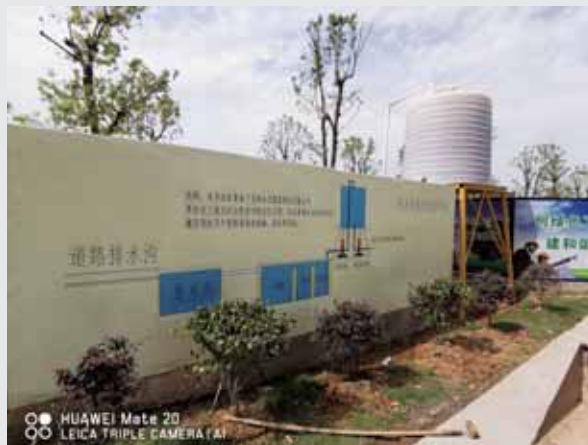
Rainwater collection system on construction site
