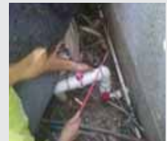
Routine maintenance of water supply equipment
