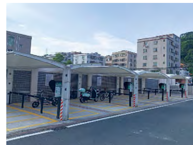
Electric Bike Charging Piles
