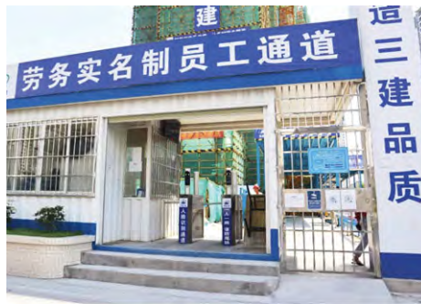
Fully enclosed site management
