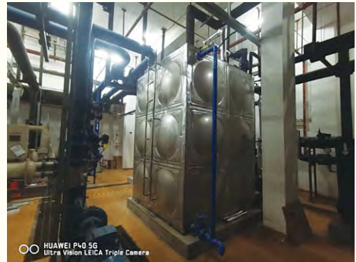
Air conditioning waste heat recovery equipment
