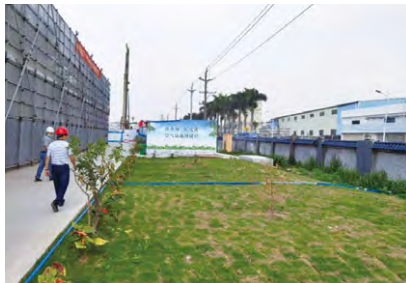
The bare soil at the construction site is covered with turf
