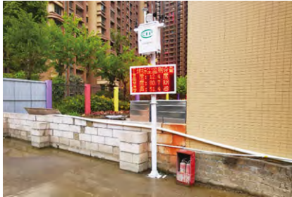
Dust detectors are installed at the construction site
