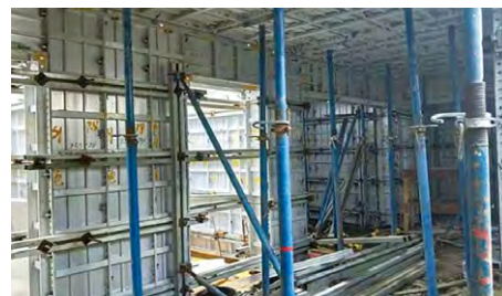
Prefabricated reusable building components on construction site
