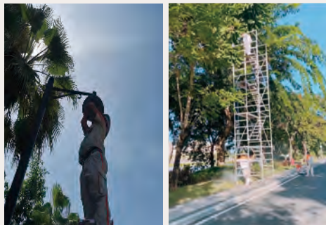
The I, II and III Phases of Clearwater Bay No. 3 project replaced corn lamps with low-energy floodlights
