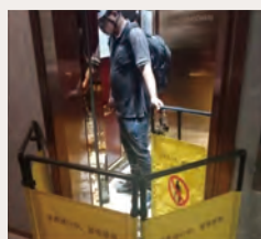
Maintenance of the Lift Operation
