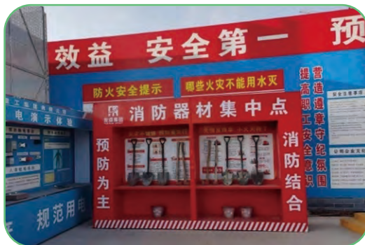
Fire Equipment Concentration Point
