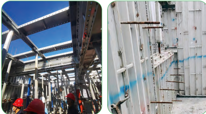
Application of Assembly Building Technology
