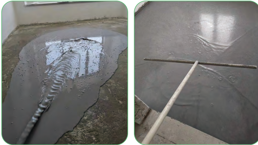
New Self-levelling Process Application
