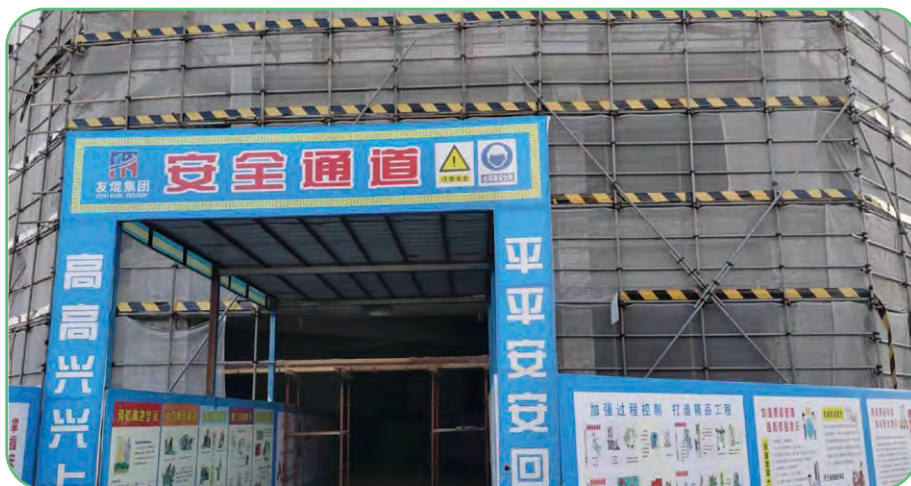
Construction Safe Passage
